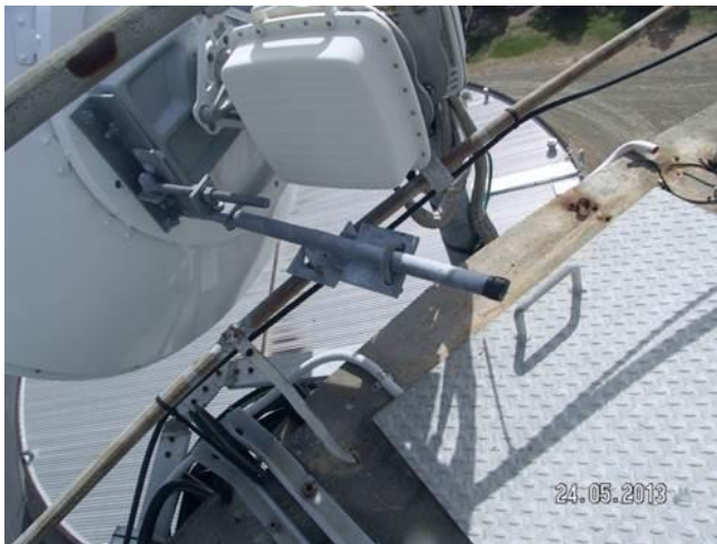
Photograph No. 3 showing blocked access hatch to water reservoir at RFNSA Site No. 4161001 located at Alexandra Hills Reservoir located at 36A Alexandra Circuit, Alexandra Hills Queensland.
