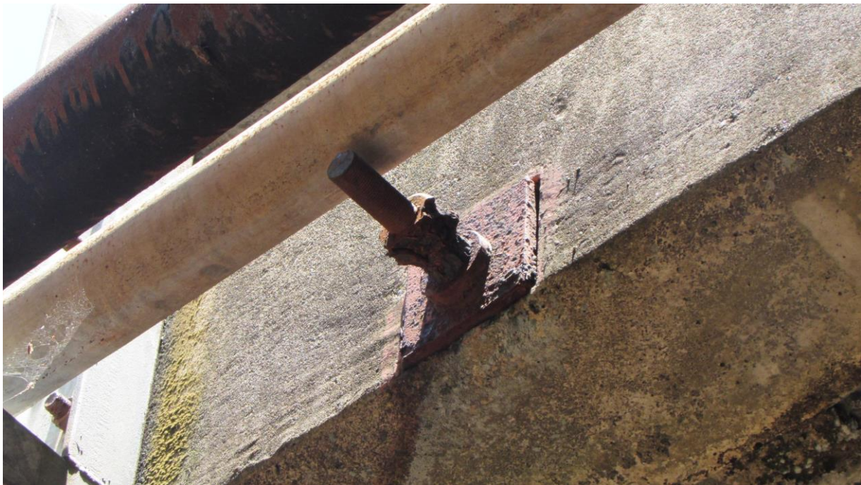
Tramway Overpass Bridge, Innisfail-Japoon Road
