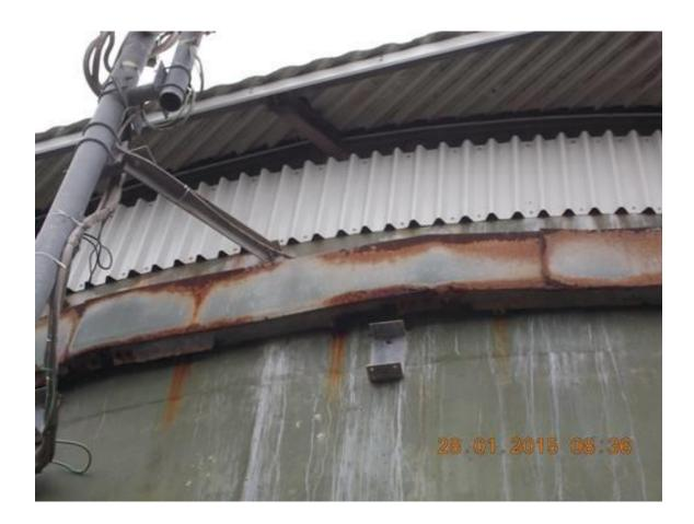
• Fixtures have been installed with little regard to the quality of the work being undertaken or its consistency, and in some cases with little to no regard to how local water utilities will be able to carry out their required maintenance operations. Please see the photograph below as an example of where this has occurred. In this instance, an access hatch could not be opened.
