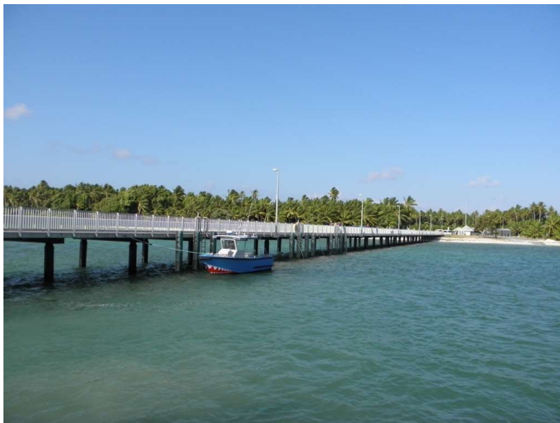
Jetty, West Island, Cocos (Keeling) Islands
