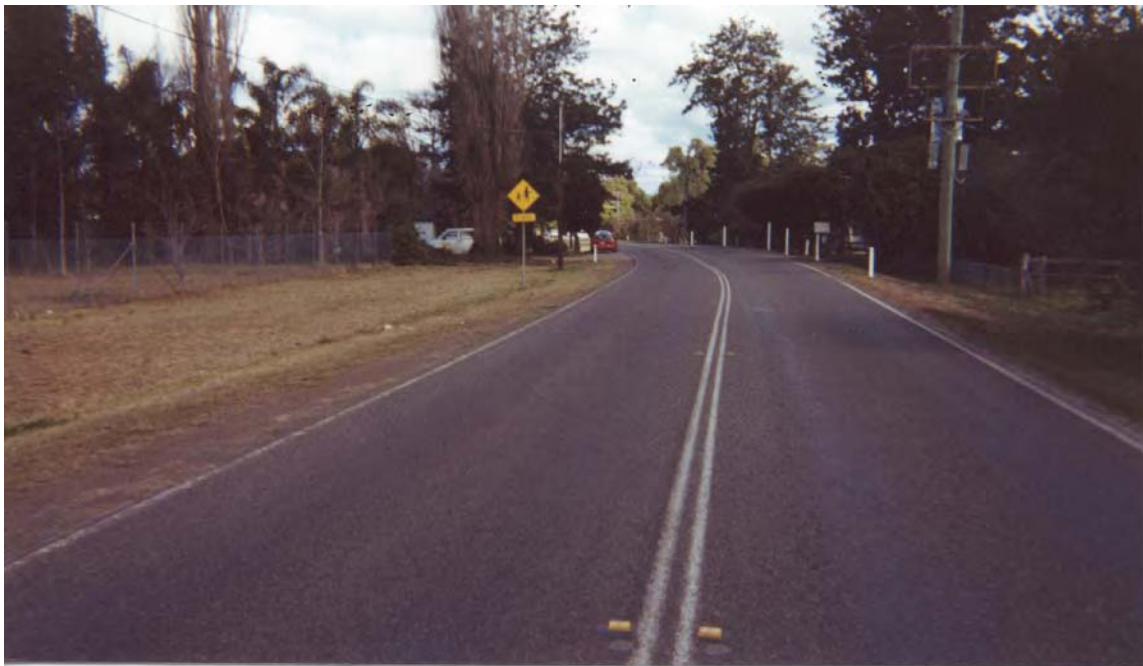
Figure 15: Castlereagh Road, NSW (south-westbound, past Springwood /road near no. 460): Treatment Site – After Installation of Treatment. Note: Wide spacing of posts due in part to driveways
