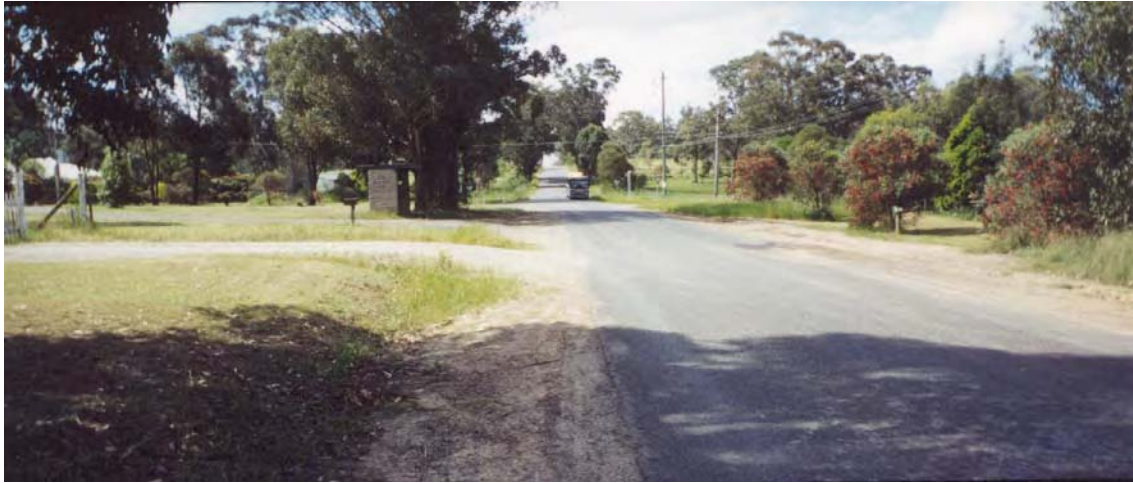
Figure 29: Old Stock Route Road at Wolseley Road, NSW: Control Site
