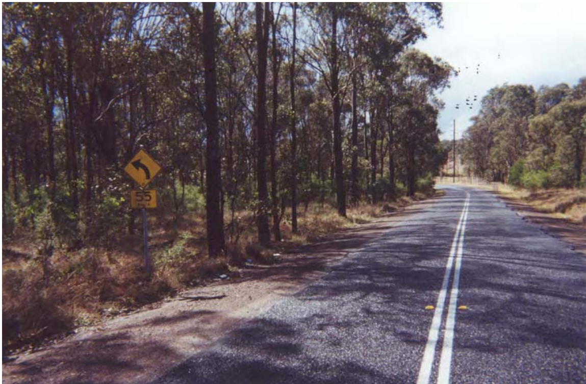
Figure 17: Scheyville Road, NSW (eastbound, past Dormitory Hill Road): Treatment Site – After Installation of Treatment. Note: Posts very close together
