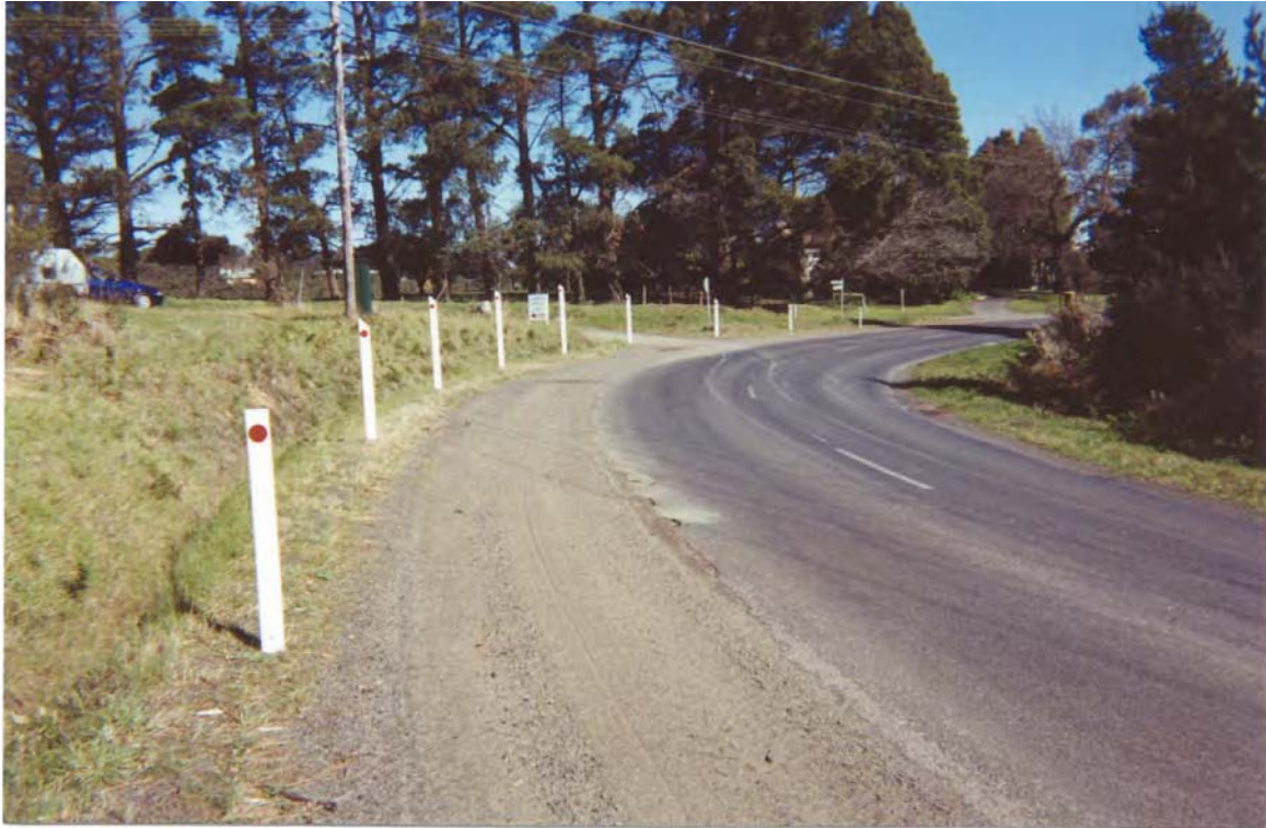
Figure 3: Gembrook Road, Victoria (southbound, opposite no. 605): Treatment Site – After Installation of Treatment
