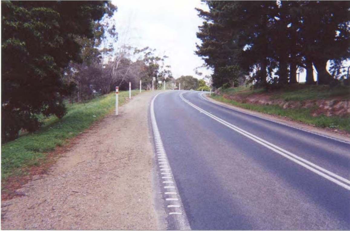
Figure 9: Harkaway Road, Victoria (southbound, past no. 186 opposite 'Melrose'): Treatment Site – After Installation of Treatment
