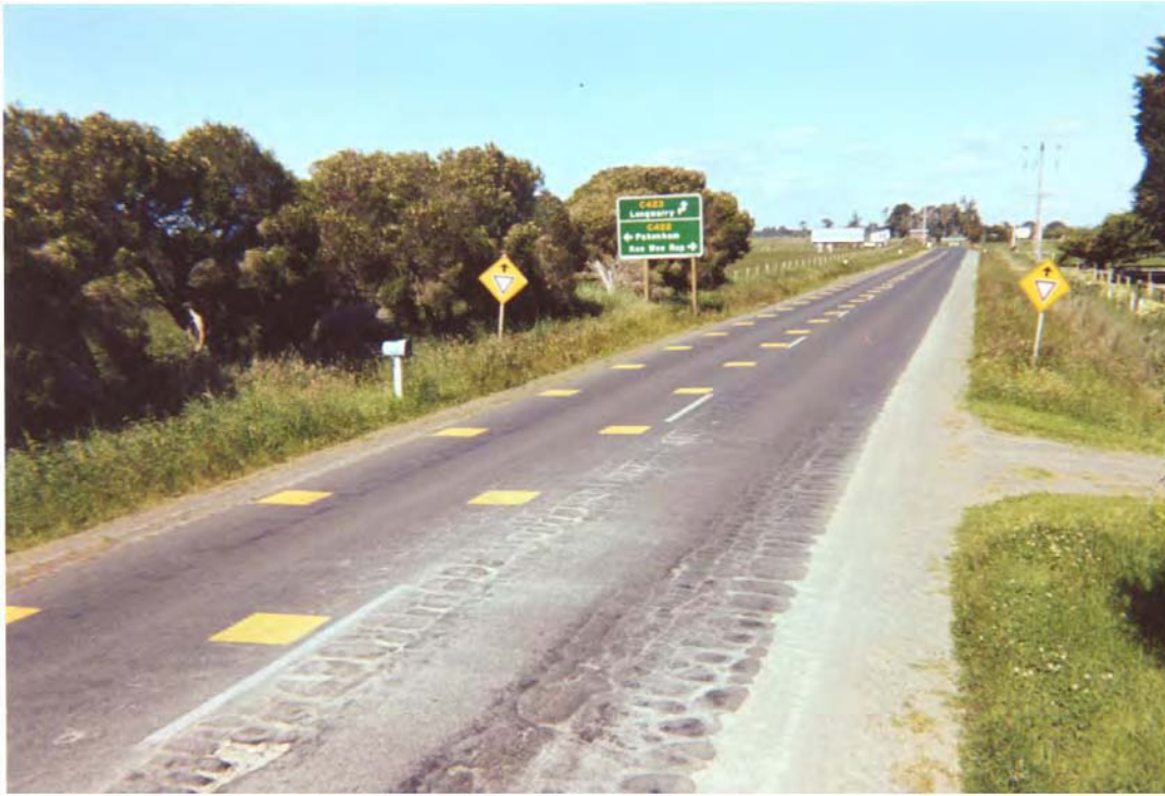
Figure 20: Ballarto Road at Koo Wee Rup Road, Victoria: Treatment Site – After Installation of Treatment
