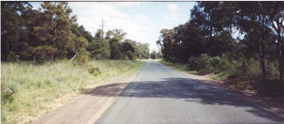
Figure 30: Old Stock Route Road at Wolseley Road, NSW: Treatment Site – Before Installation of Treatment
