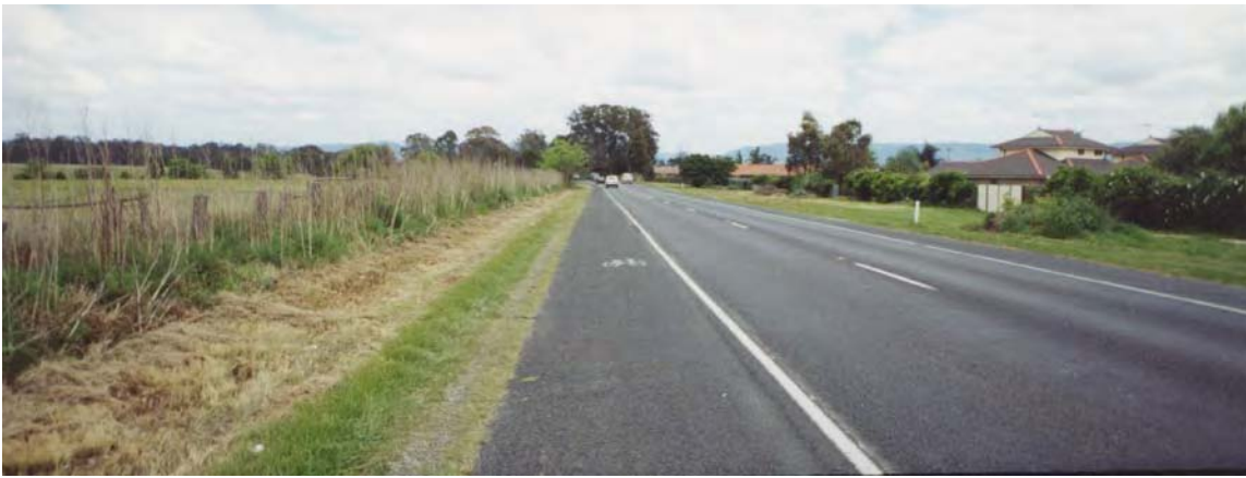
Figure 13: Castlereagh Road, NSW (south-westbound, between Inalls Road and Drift Road): Control Site
