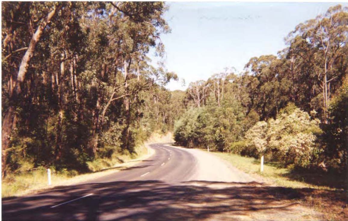
Figure 4: Pakenham Road, Victoria (southbound, south of Paternoster Road): Control Site
