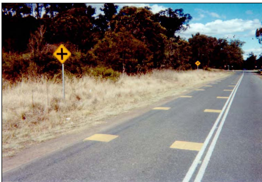
Figure 3.2: Typical Intersection Treatment
