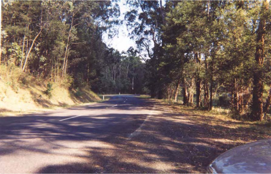
Figure 5: Pakenham Road, Victoria (southbound, north of Mann Road): Treatment Site – Before Installation of Treatment
