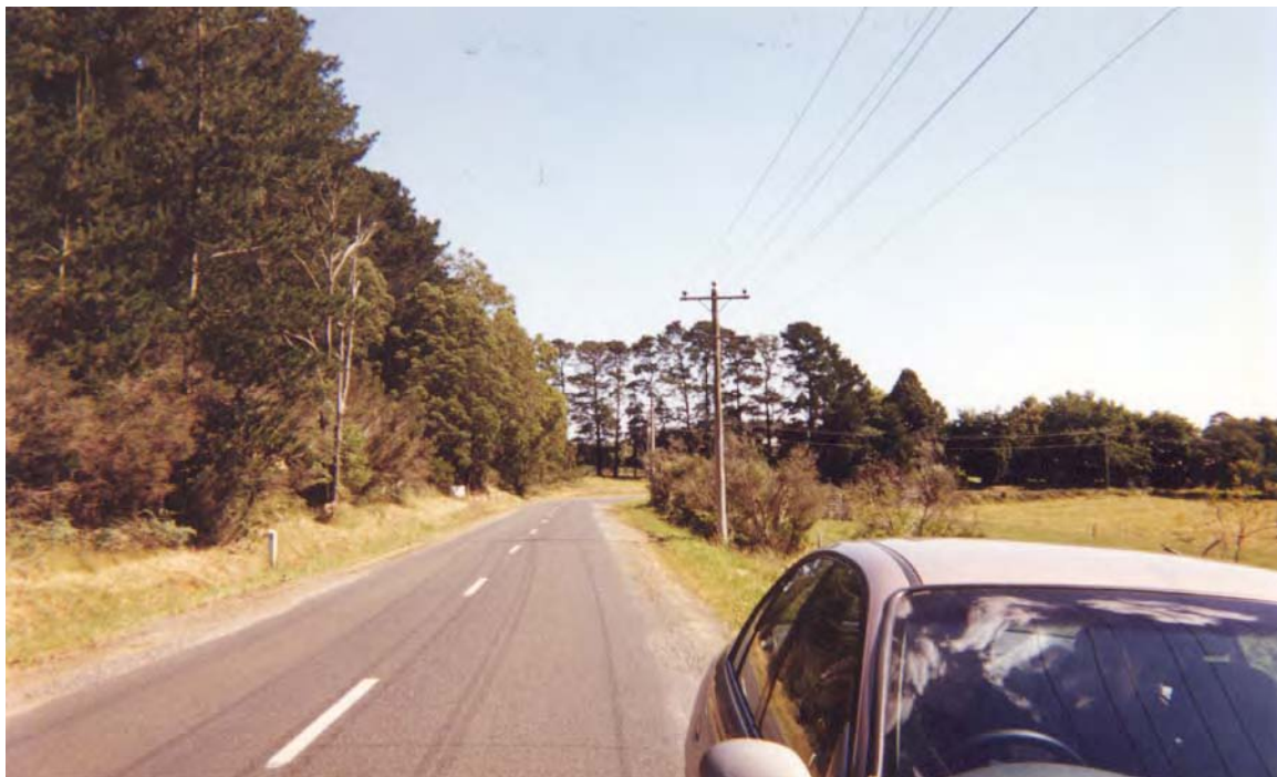
Figure 2: Gembrook Road, Victoria (southbound, opposite no. 605): Treatment Site – Before Installation of Treatment
