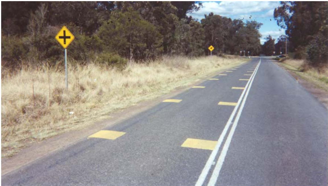
Figure 31: Old Stock Route Road at Wolseley Road, NSW: Treatment Site – After Installation of Treatment
