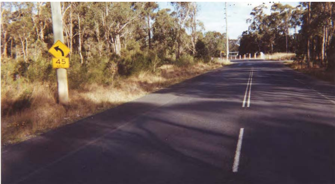
Figure 12: The Driftway, NSW (southbound, at Bonner Road): Treatment Site - After Installation of Treatment
