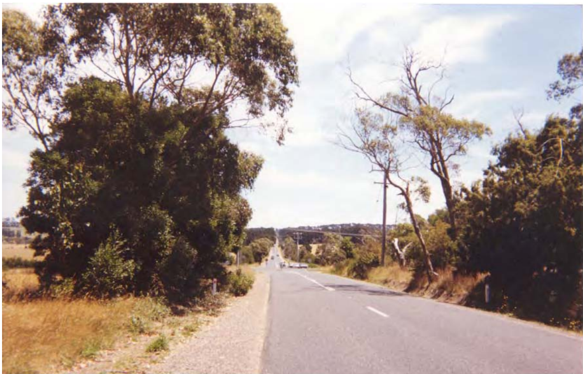
Figure 22: Bittern Dromana Road at Balnarring Road, Victoria: Treatment Site – Before Installation of Treatment
