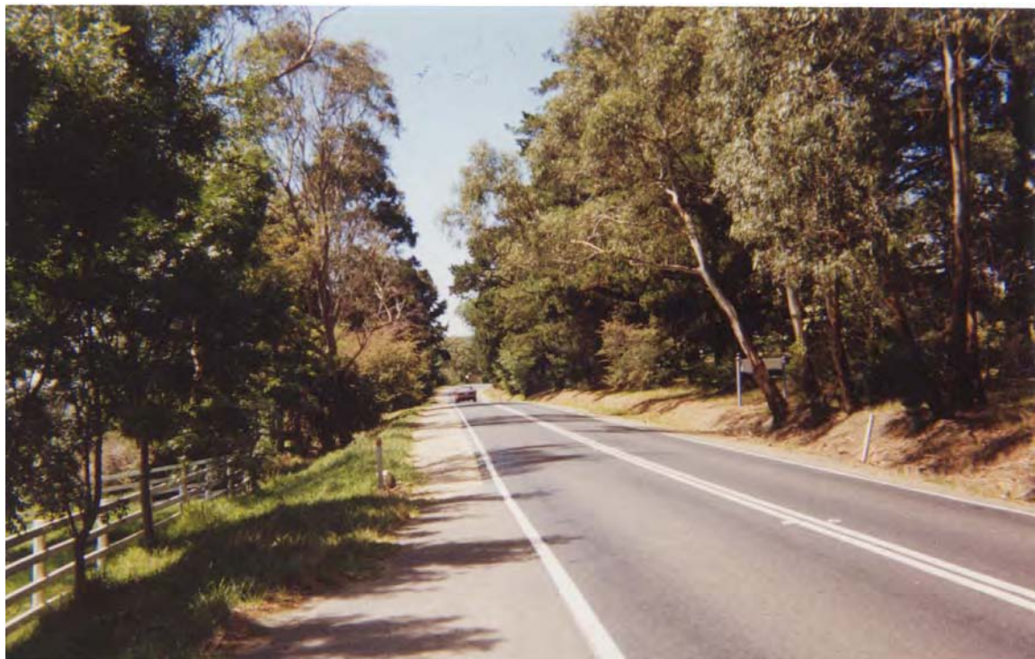
Figure 8: Harkaway Road, Victoria (southbound, past no. 186 opposite 'Melrose'): Treatment Site – Before Installation of Treatment
