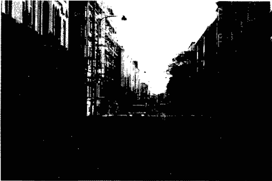
Photo 3: Drottninggatan (from east). (Inner road, 50 km/h speed limit) Note: Narrowed pavement (2 traffic lanes). Tree planting on one side to give narrow visual appearance (both sides were desired, but could not be accommodated).
