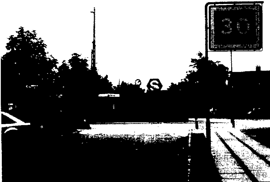
Photo 13: Herlev (suburb of Copenhagen). (Entry to local road (near railway), 30 km/h advisory speed limit) Note: Roadway narrowing with gateway appearance. Pavement rises onto cobble stones. Posts and shrubs.
