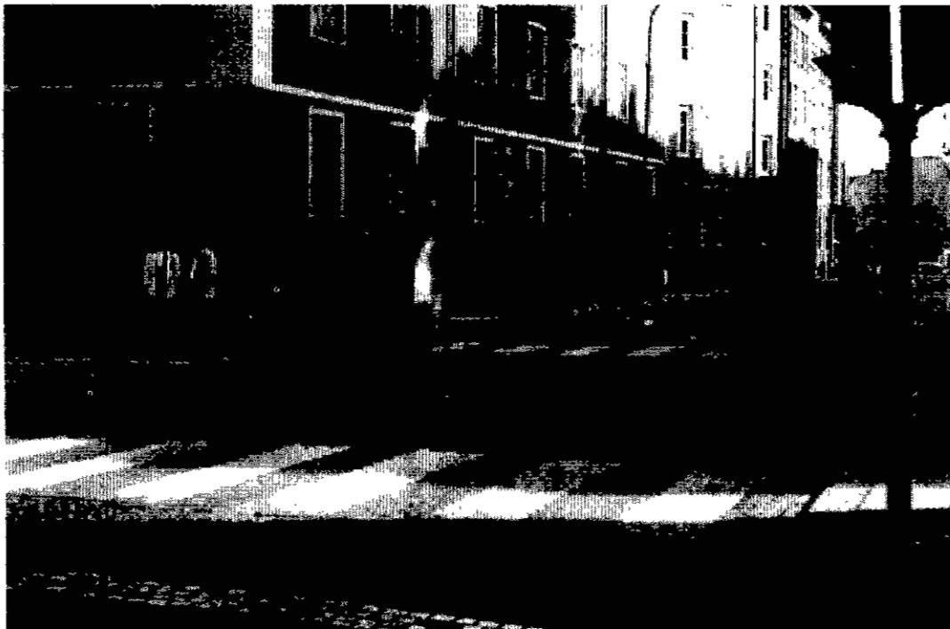
Photo 4: Drottninggatan (at T intersection). (Inner road, 50 km/h speed limit) Note: Cobble stones for motor traffic. Contrasting paving bricks on pedestrian crossings. Different paving bricks for bicycle paths.
