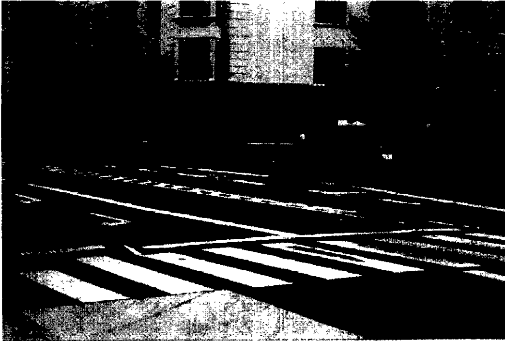
Photo 12: Strandvejen, at Hellerupvej. (Traffic road, 50 km/h speed limit) Note: Closure of minor street entering near major intersection. Road reserve of closed street allows provision of parking bays.
