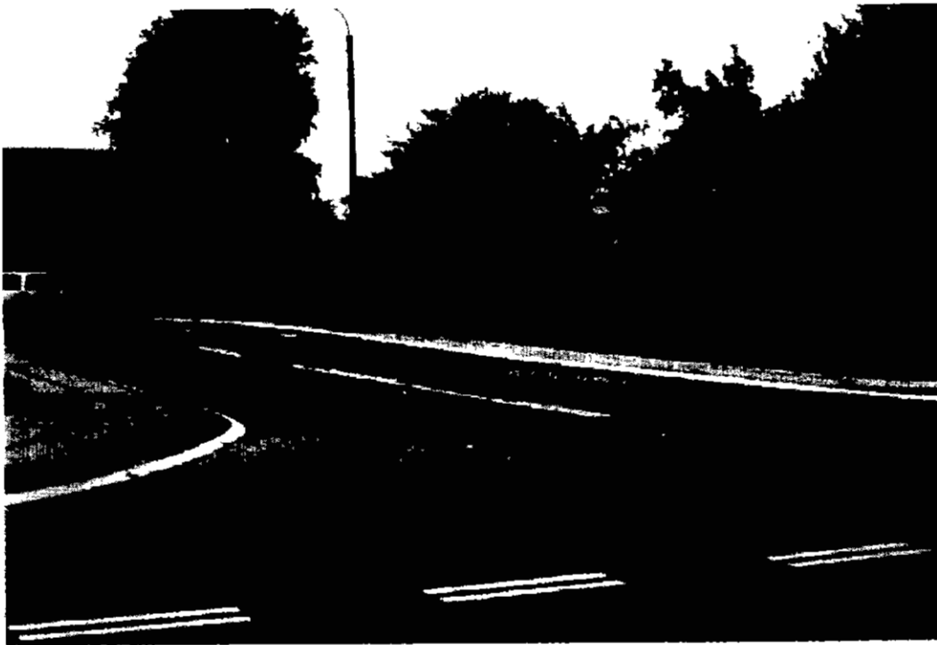
Photo 19: Hareskoven (suburb of Copenhagen). (Traffic road (through residential area), 40 km/h speed limit) Note: Narrow pavement (2 traffic lanes). Heavy trucks prohibited. Parking bays. Raised paving bricks (hump) at entry. Frequent use of circular humps along route (not shown).
