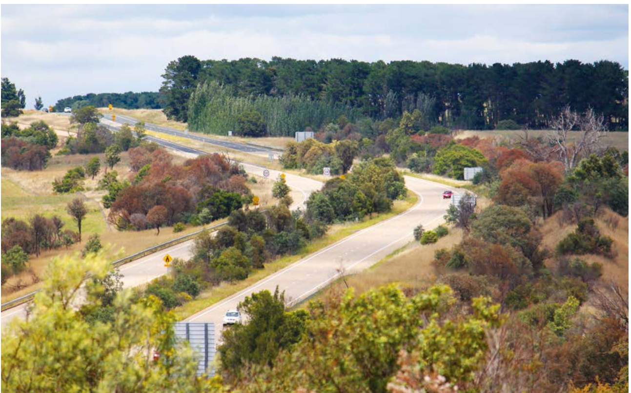
Existing Barton Highway dual carriageway, south of the Hume Highway, near Yass
