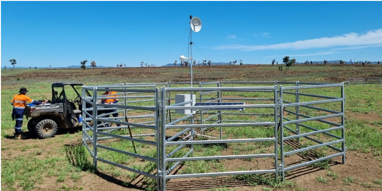
Figure 9 – Starlink + WiFi covering 250 m radius with voice, text, and data services
