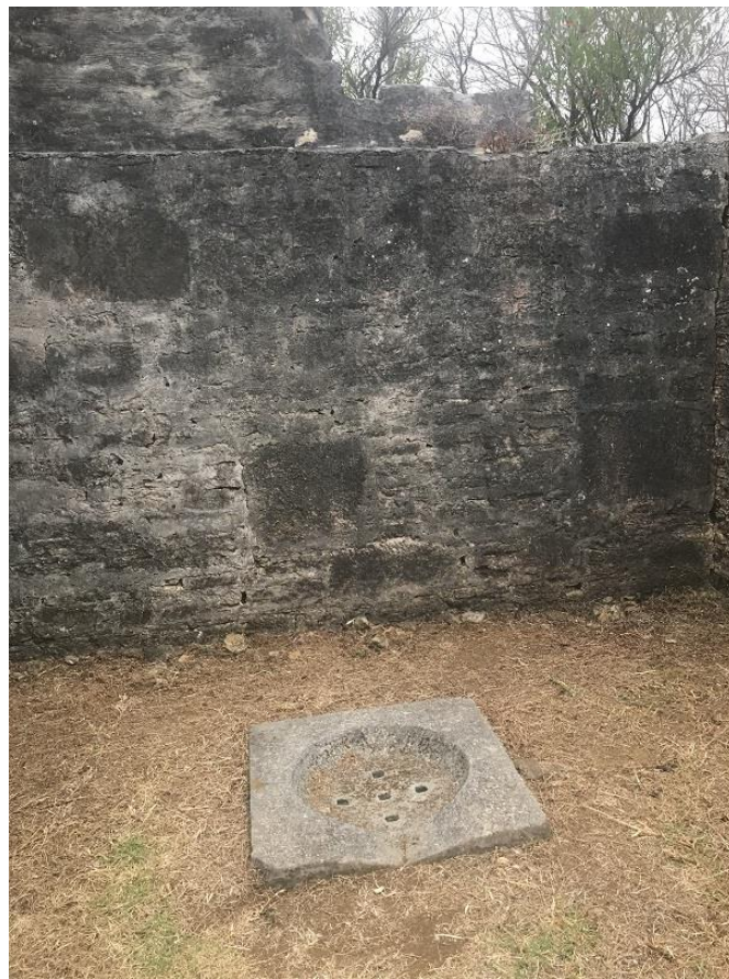
Figure 10: Surviving stone drain in southern ground floor interior room, 2019. Photo: Australian Government, 2020
