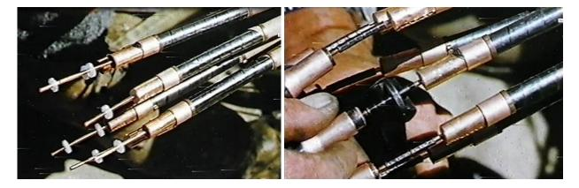
The above left picture shows the coax cable tubes with their polyester spacers around the centre conductors and on the right showing the centre conductor being crimped in a sleeve (as also was the outer tube (9.525 mm) with a steel inner sleeve shown near his thumb). These cables were dry gas pressurised to try and minimise water ingress as these tubes and the interstice quads were all paper-insulated.
