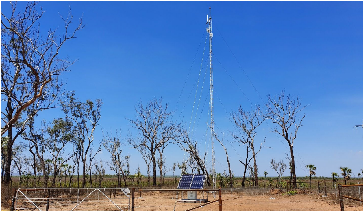
Figure 10 - LoRa IoT base station in remote Northern Territory
