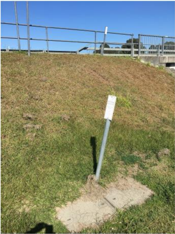
Pit location at the end of Larry Storey Bridge
