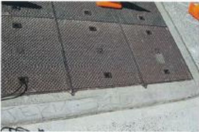
Photo 5 - Access manhole at northern end of bridge
