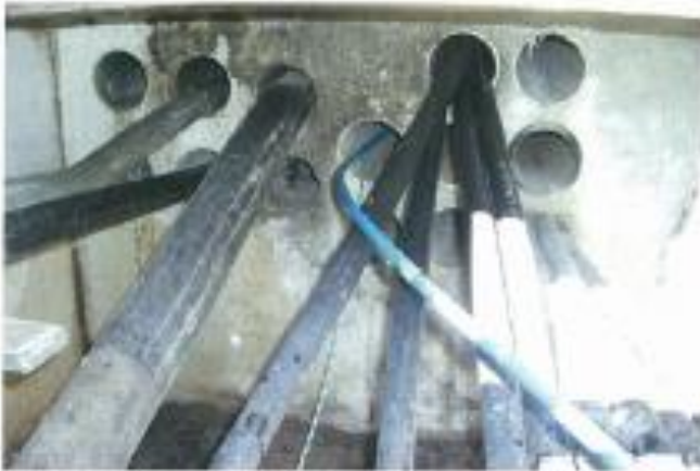
Photo 1 - Nest of telecommunications ducts located in bridge.
