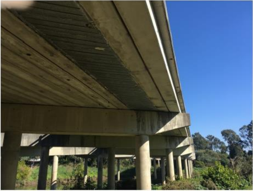
Duct space underneath Larry Storey Bridge
