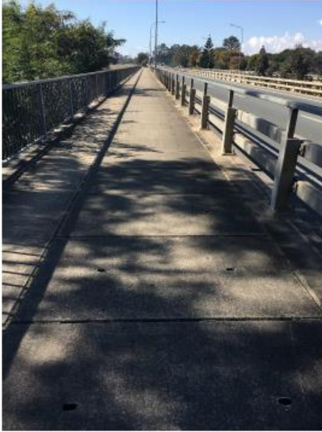
Footpath above duct space on Larry Storey Bridge
