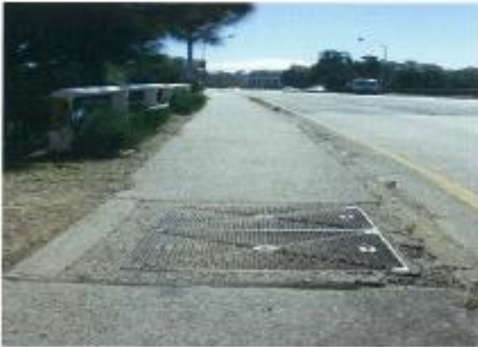
Photo 4 - Access manhole at southern end of Bridge
