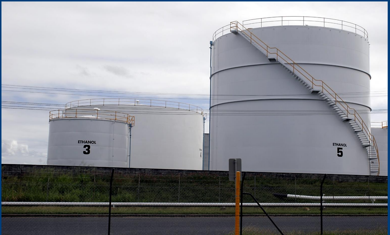
Ethanol Storage Tanks at Mackay Harbour
