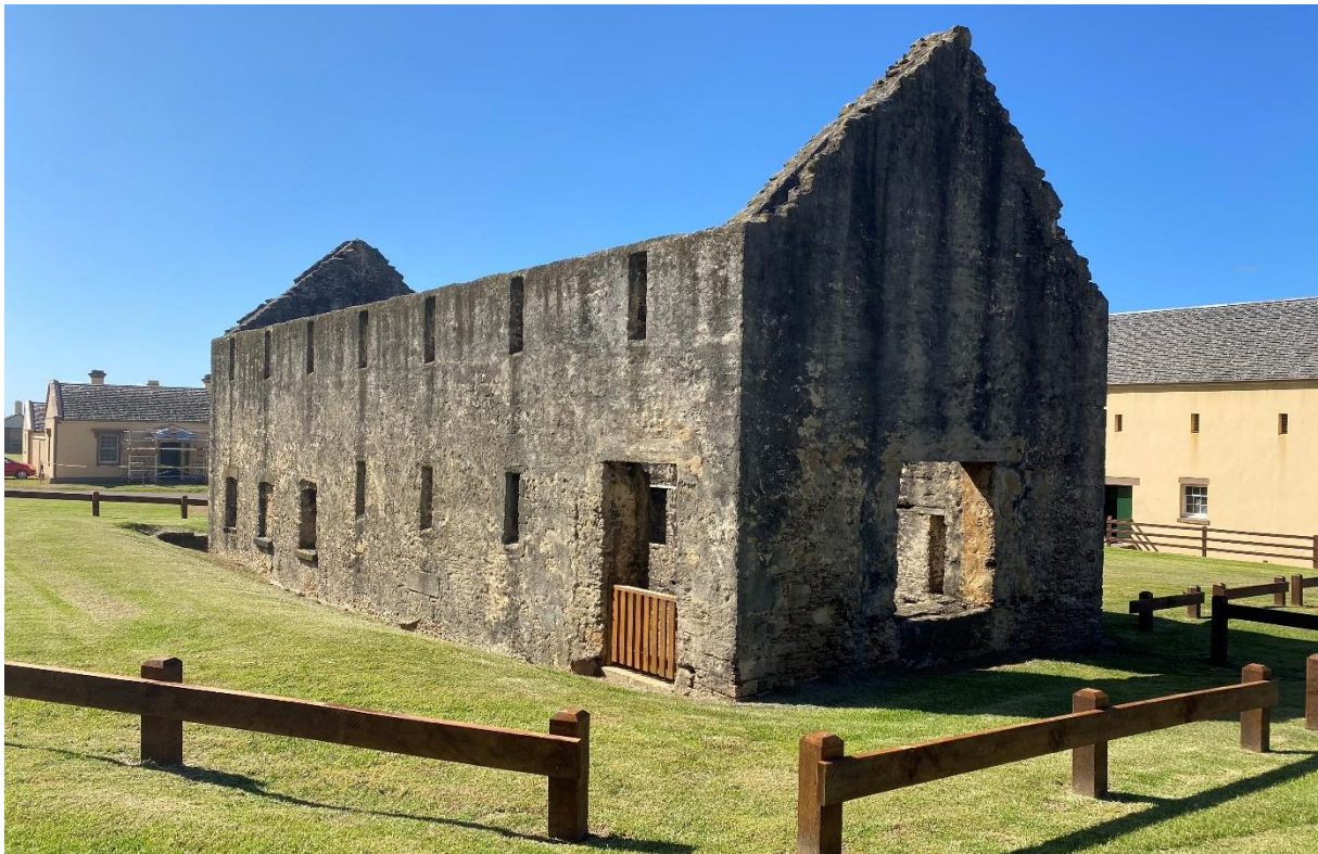
Figure 7.8 Ruins of the Crankmill, made of local rubble calcarenite limestone, 2021
