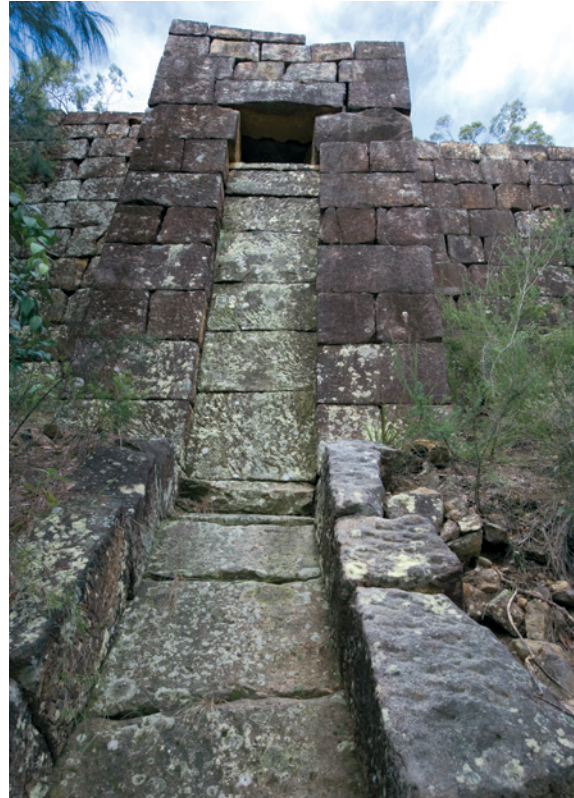
Old Great North Road (Department of the Environment and Energy)
