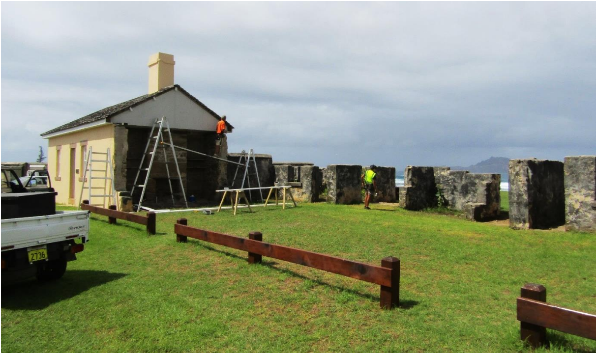
Figure 7.7 Works in progress at the blacksmith's shop, known locally as 'Munna's', 2022.
