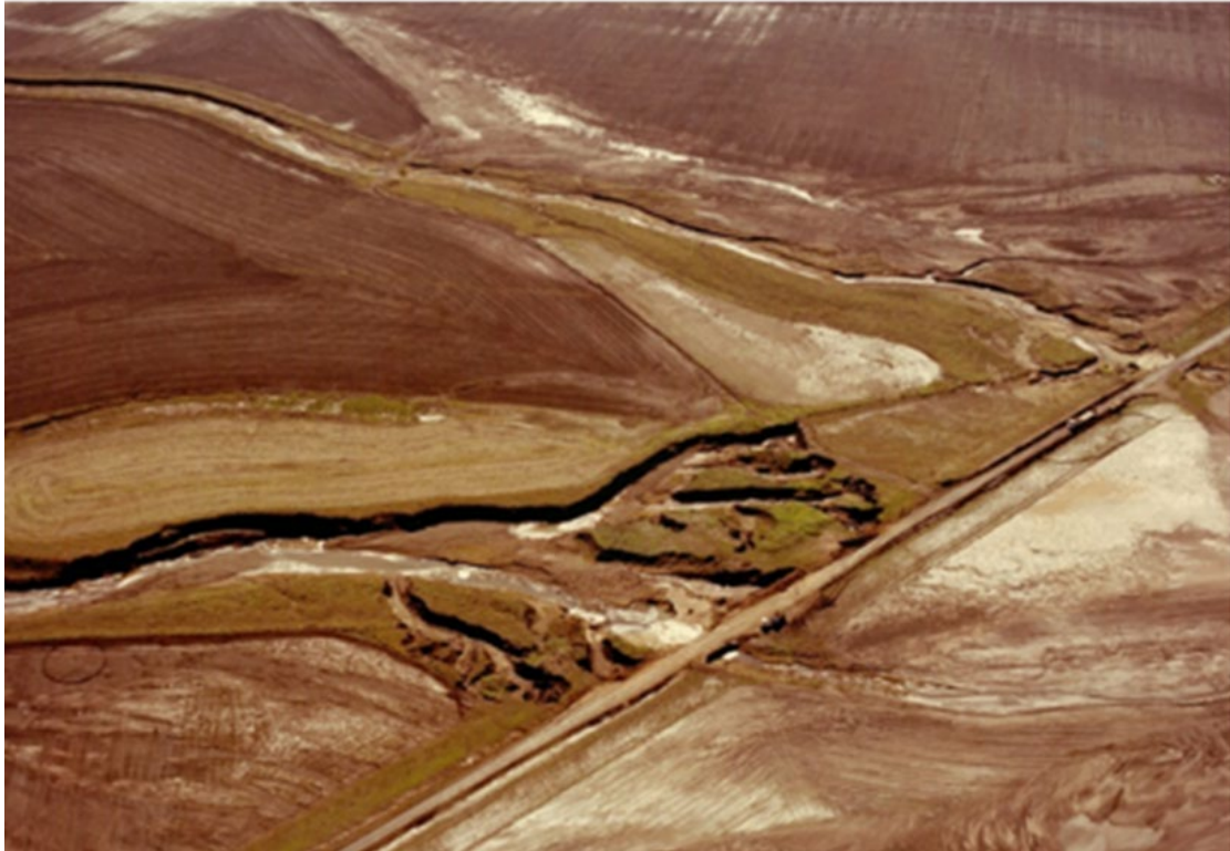
Figure 3: Two gullies formed downstream of road crossings, Linthorpe Creek, Toowoomba – Cecil Plains Road.
