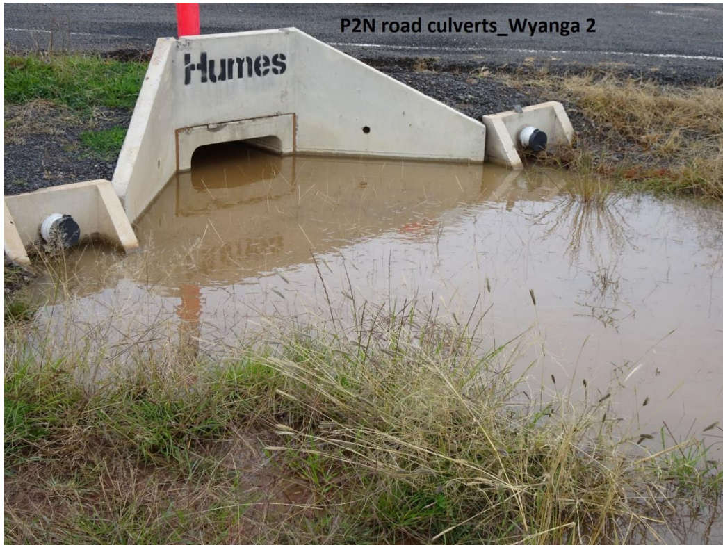
P2N Example of Road-Rail Culverts Installed below Flow Level
