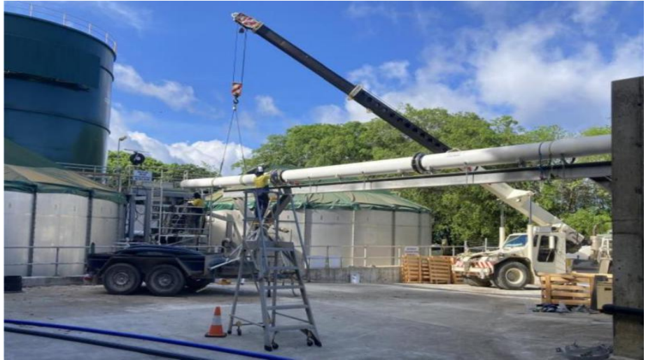
Image: In action, clarifier overhead pipe replacement
