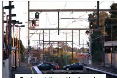
Previous station and level crossing
