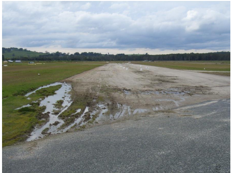
Intersection Runways 02/44 and 18/36, looking north
