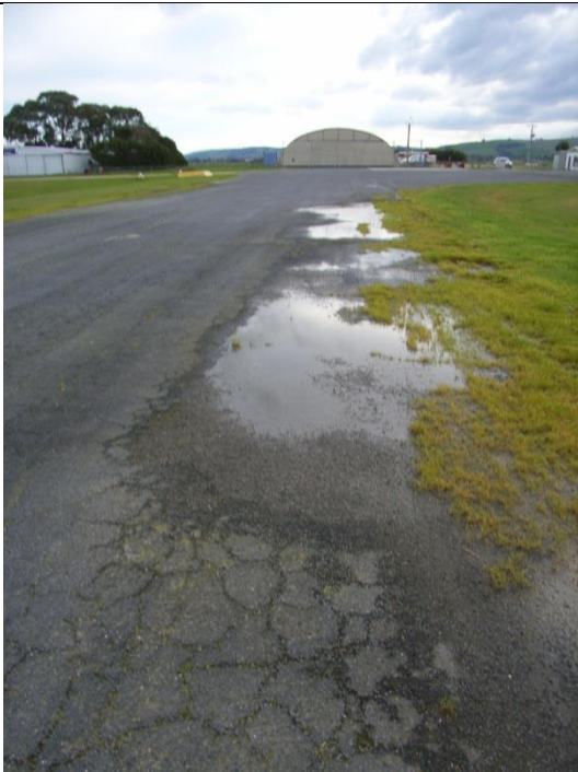
Taxiway A, looking west
