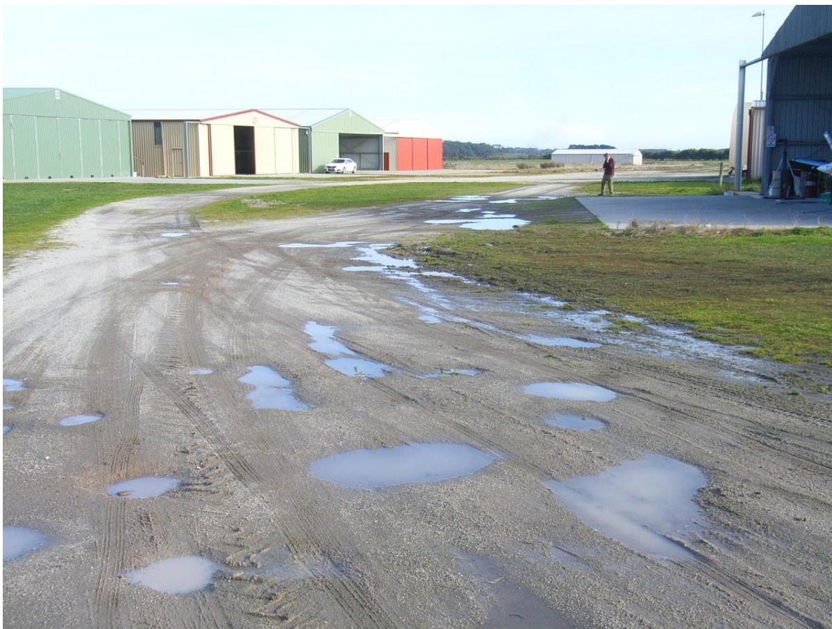
Taxiway D looking South
