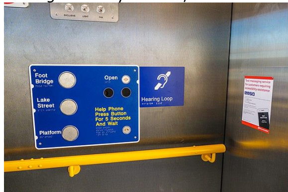
Lift car that carries audio announcements via hearing loop, Yeronga Railway Station, Brisbane.
