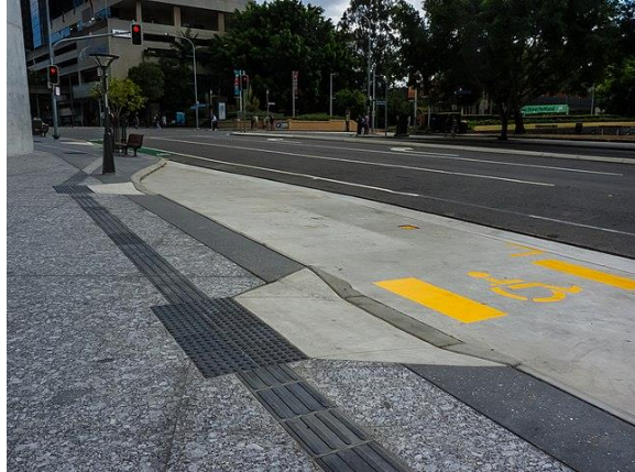
Passenger and commercial loading zone with kerb ramp, Russell St, South Brisbane.
