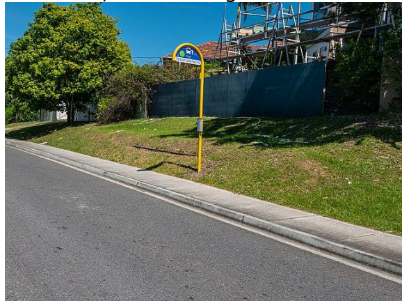
Boarding point constrained by crossfall and road gradient, Edinburgh Castle Rd, Wavell Heights.
