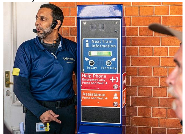
Platform help phone not equipped with hearing loop, South Brisbane railway station.
