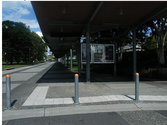
Passenger loading zone at grade with footpath, Powerhouse Theatre, New Farm, Brisbane.
