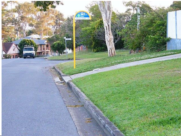
Boarding point unsealed and constrained by crossfall, Piccadilly St, Geebung.
