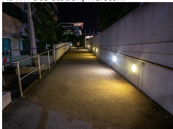
Light pools and glare on access path, RBWH bus station, Herston.
