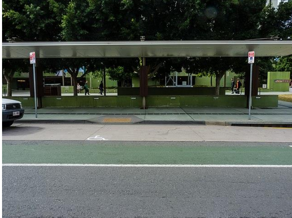
Passenger loading zone with kerb ramp, Stanley Place, South Brisbane.
