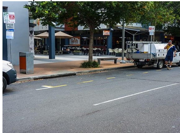
Passenger and commercial loading zone lacking kerb ramps, Little Stanley St, South Brisbane.
