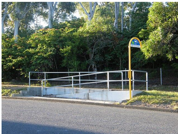
Boarding point constrained by crossfall, Ellison Rd, Geebung.
