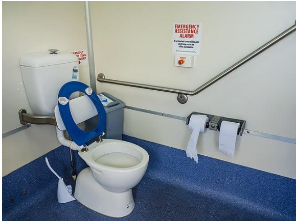
Ferry emergency call button on wall adjacent to pan but no lower call button.
