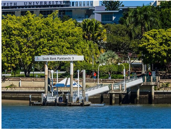
South Bank 3 ferry terminal and pontoon waiting area.
