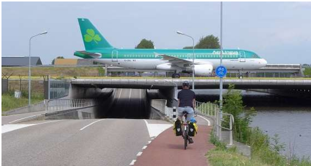
Schiphol Airport taxiway underpass with bike path
