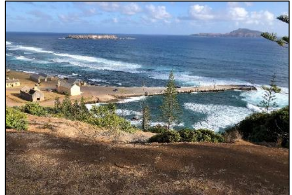
Figure 1-24 View looking south-east from Flagstaff Hill to Kingston Pier, Phillip and Nepean Islands (Source: Advisian 2020).
