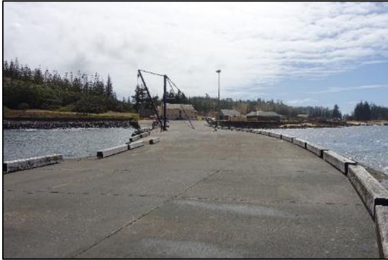
Figure 1-20 View looking north at Kingston Pier (Source: Advisian 2020).
