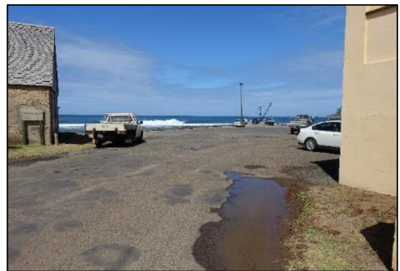
Figure 1-7 View looking south-west to the hardstand area at Kingston Pier (Source: Advisian 2020).
