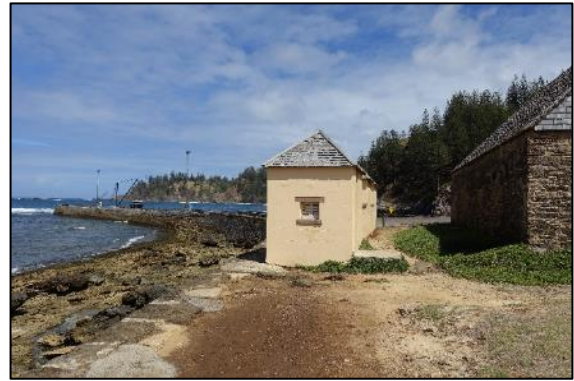
Figure 1-9 View looking west at the stone seawall to the Boatsheds, Flaghouses and Kingston Pier (Source: Advisian 2020).
