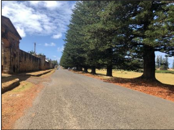
Figure 1-2 View looking east along Quality Row (Source: Advisian 2020).
