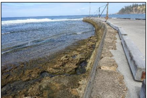
Figure 1-11 View of the eastern side of Kingston Pier (Source: Advisian 2020).
