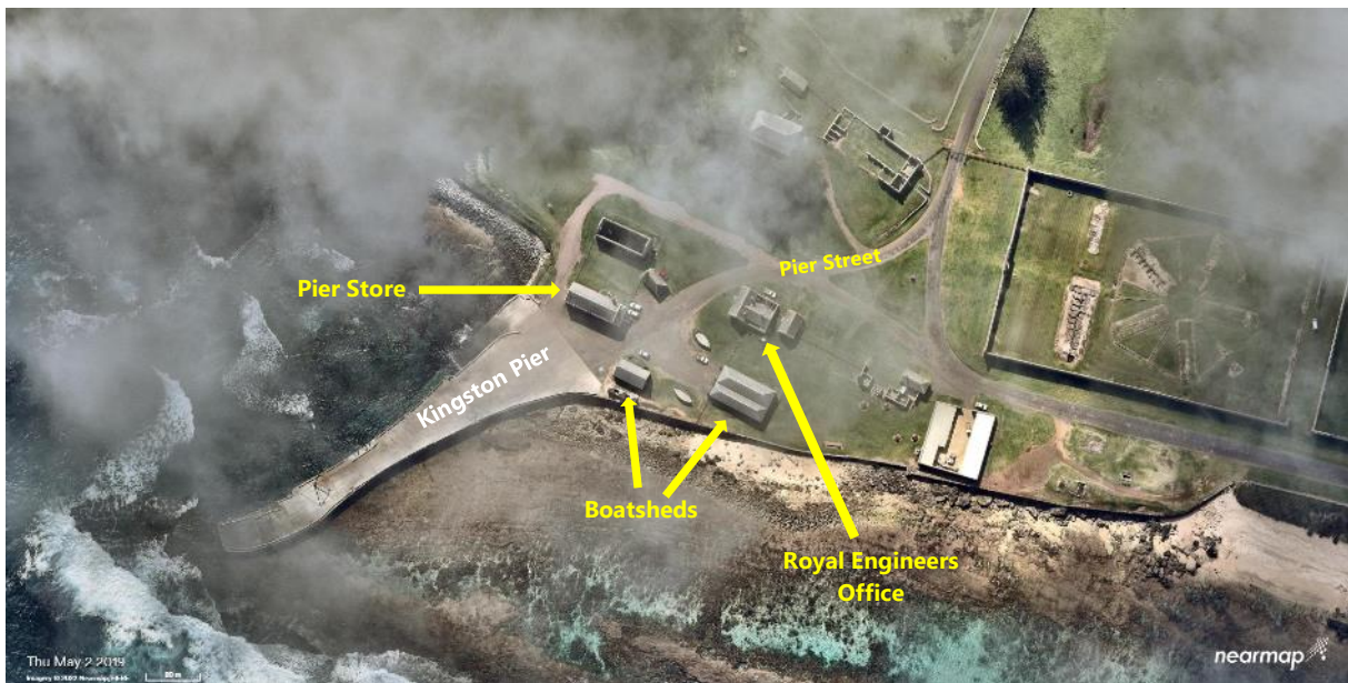
Figure 2-1 Nearby sensitive receivers to Kingston Pier (Source: Nearmap 2022).
