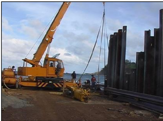
Figure 3-1 Installation of steel sheet piling.
