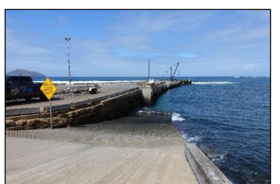
Figure 1-13 View of the western side of Kingston Pier (Source: Advisian 2020).
