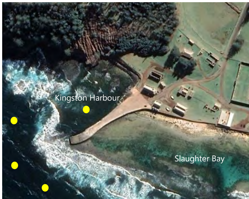
Figure 6-3 Potential turbidity baseline and construction monitoring locations (handheld measurements) inside and outside Kingston Harbour.
