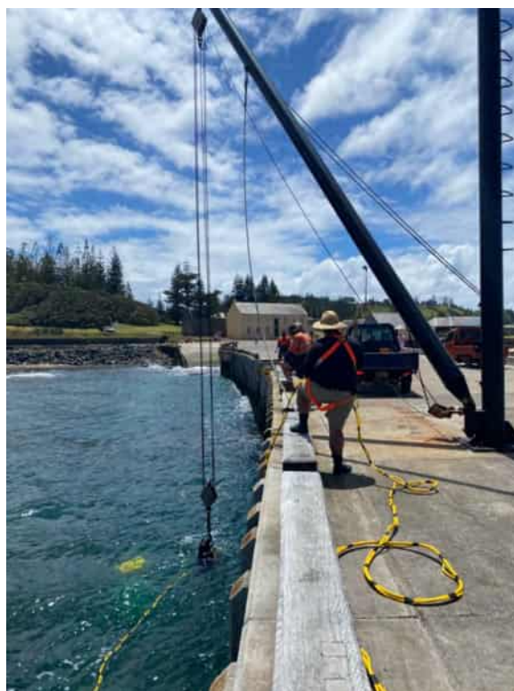
Figure 19: Method of extracting sediment boxes using Pier derrick. (Image taken 11 November 2020).
