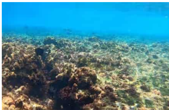
Figure 74: Rock platform running out from the southern end of Kingston Pier. A large fissure or crack is at bottom left. (Image taken from video 201117_End Kingston Pier survey JM, 00:12).
