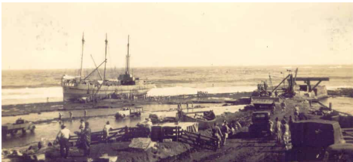
Figure 11: Ronaki IX-94 run aground on reef immediately east of Kingston Pier. Salvage efforts underway. Note the Pier is visible in the right of image. 41
